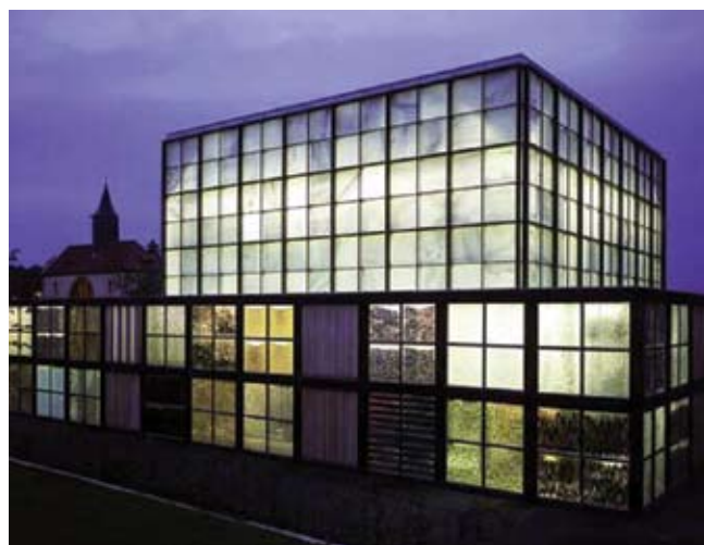
The marble-and-glass panels can be appreciated both inside and outside the structure.
